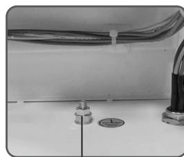
Earthing screw (PE)
